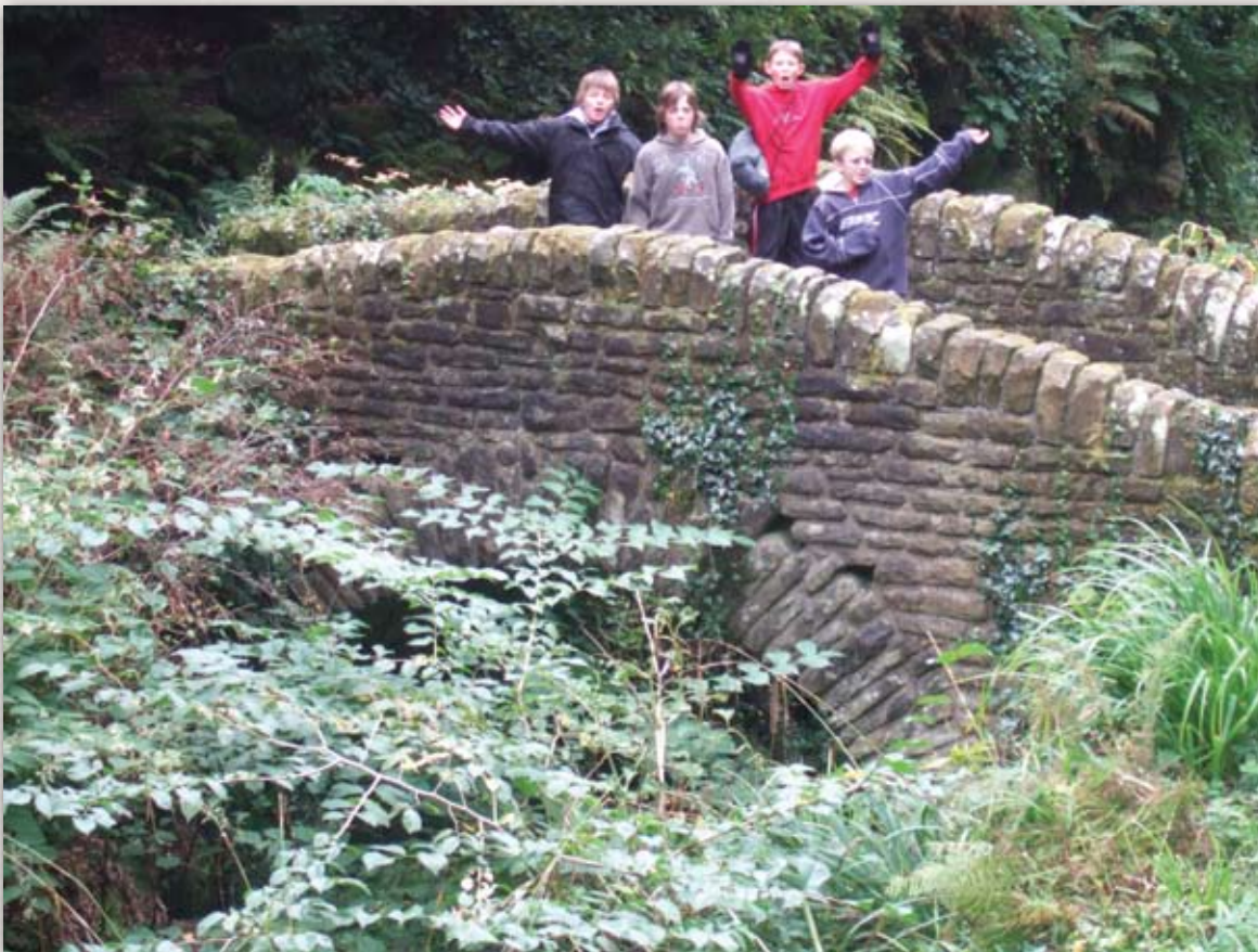
^ The Scouts visiting an example of an arch bridge.
